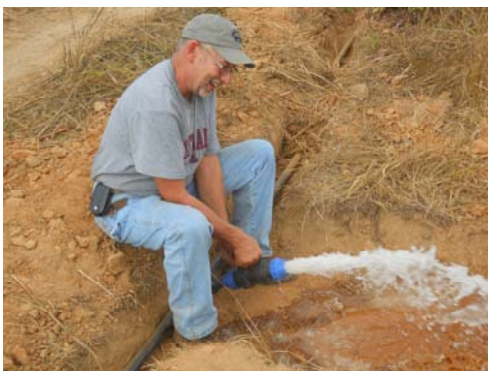
Paul testing the water pressure
